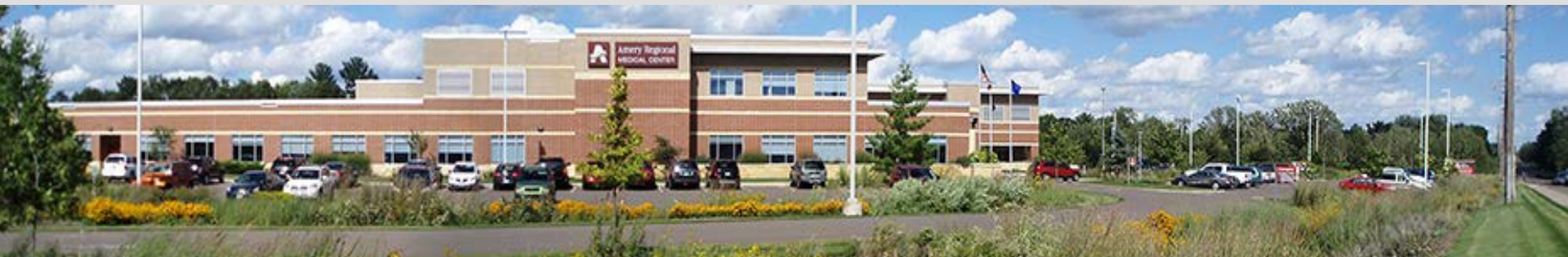
Site accommodates many different techniques
